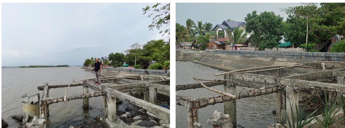
Figure 15. Beams of a damaged shelter near Masao Port, which according to the locals, was washed away by a storm surge.
