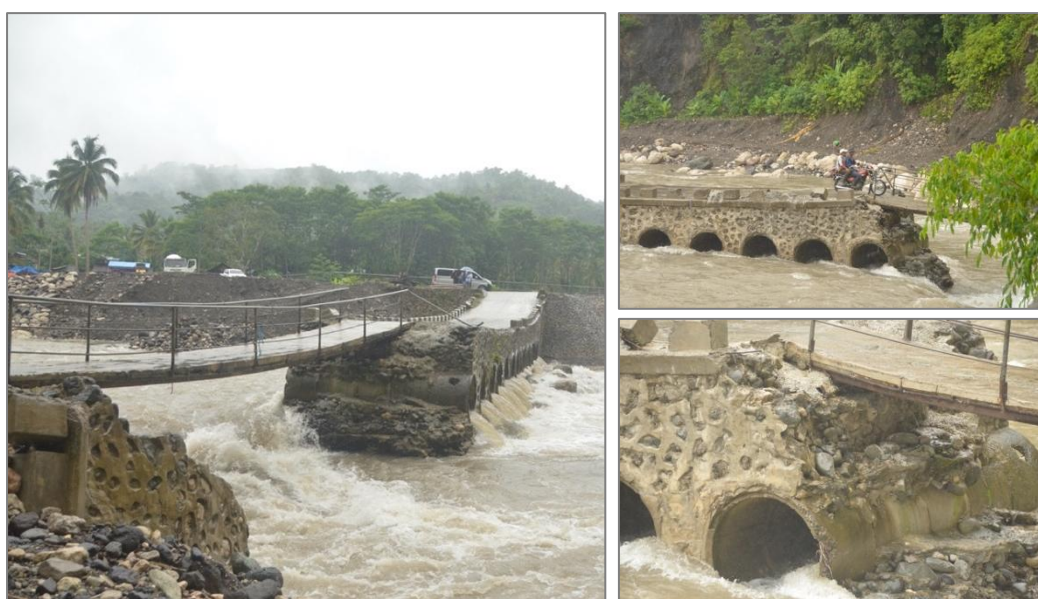
Figure 27. Bridge in Barangay Anticala that was destroyed by logs, boulders, and various debris carried by a flashflood when Typhoon Odette rampaged in December 2021.
